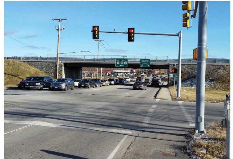
West Street at Rte 9 southbound on-ramp looking east
